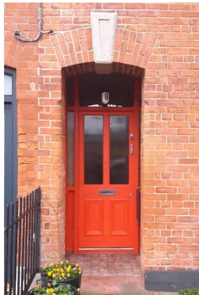
No.8 – Repair of Historic Door - 2021
