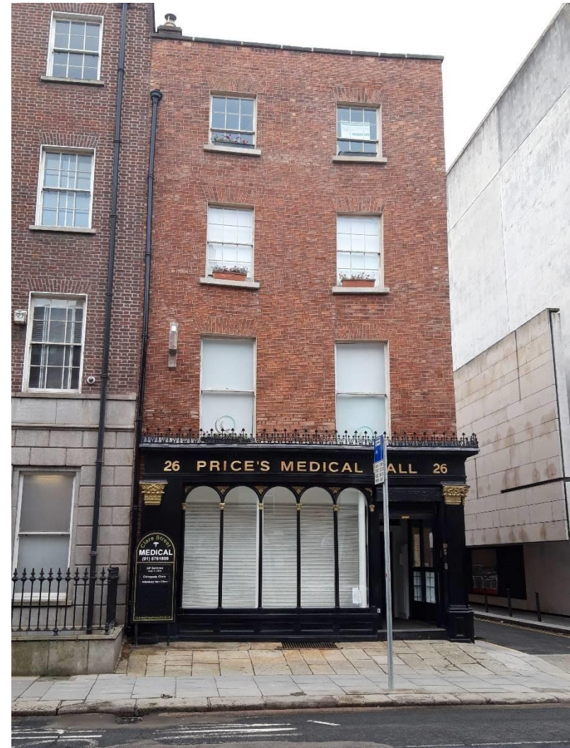
Repointing of brickwork – HSF funding 2023
