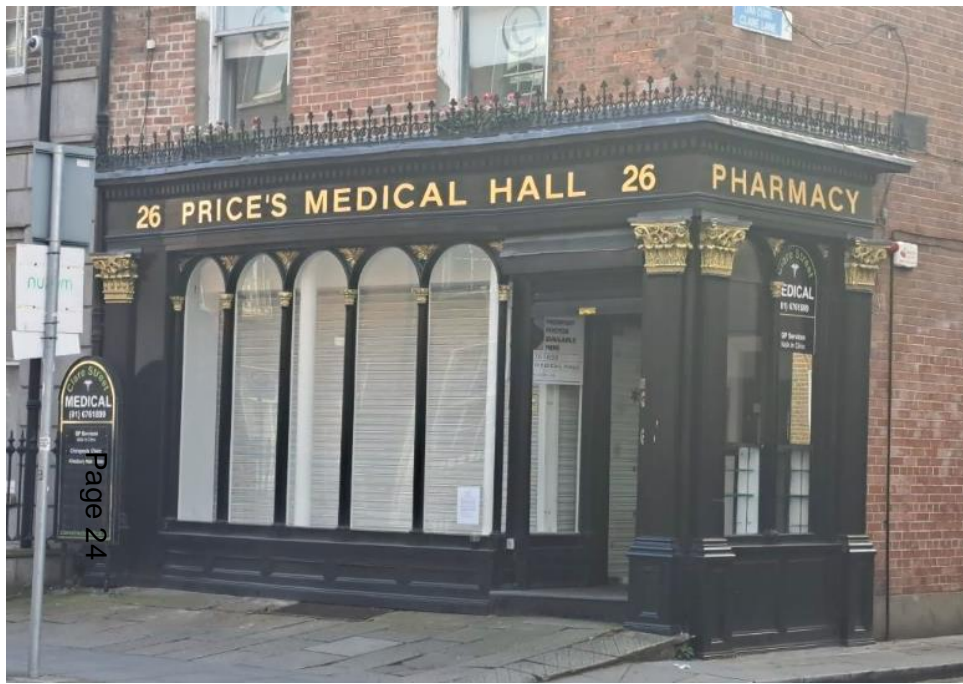
Repair of Victorian shopfront – BHIS 2020 & HSF funding 2021
