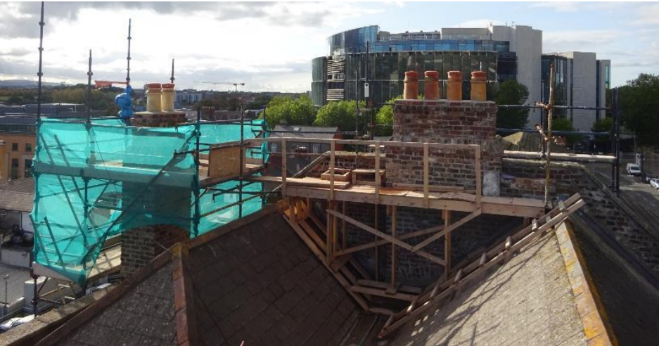
Chimneystacks & Roof Repair 2020
